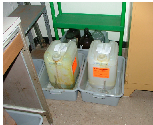
6. Example of a main accumulation area, this one is located in the Chemistry prep room
